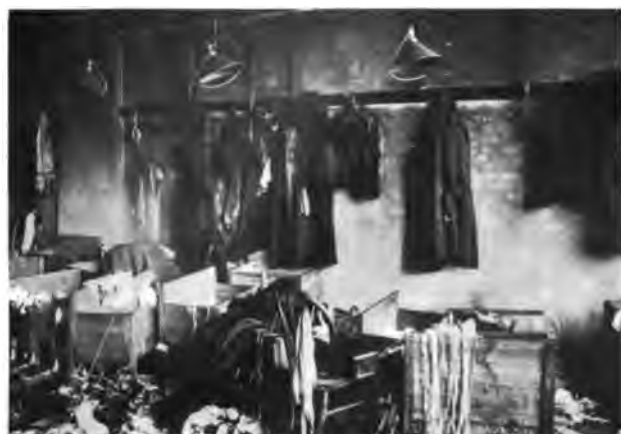
Fig. 3. Clothes Room in Building shown in Fig. 2 after Fire.*
